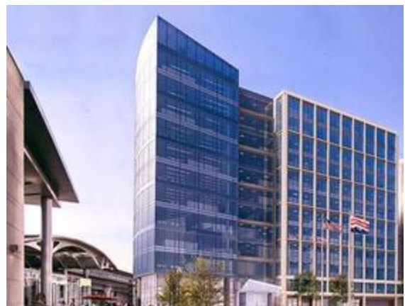
StonebridgeCarras broke ground Monday on a 345,000-square-foot spec development in the District's NoMa neighborhood.
